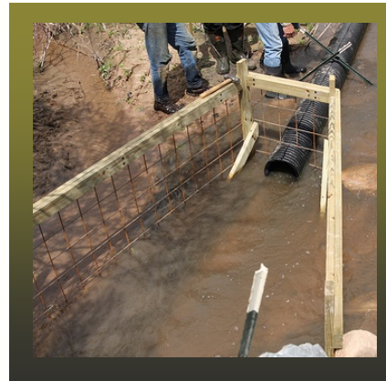
Culvert Guard Fence.
